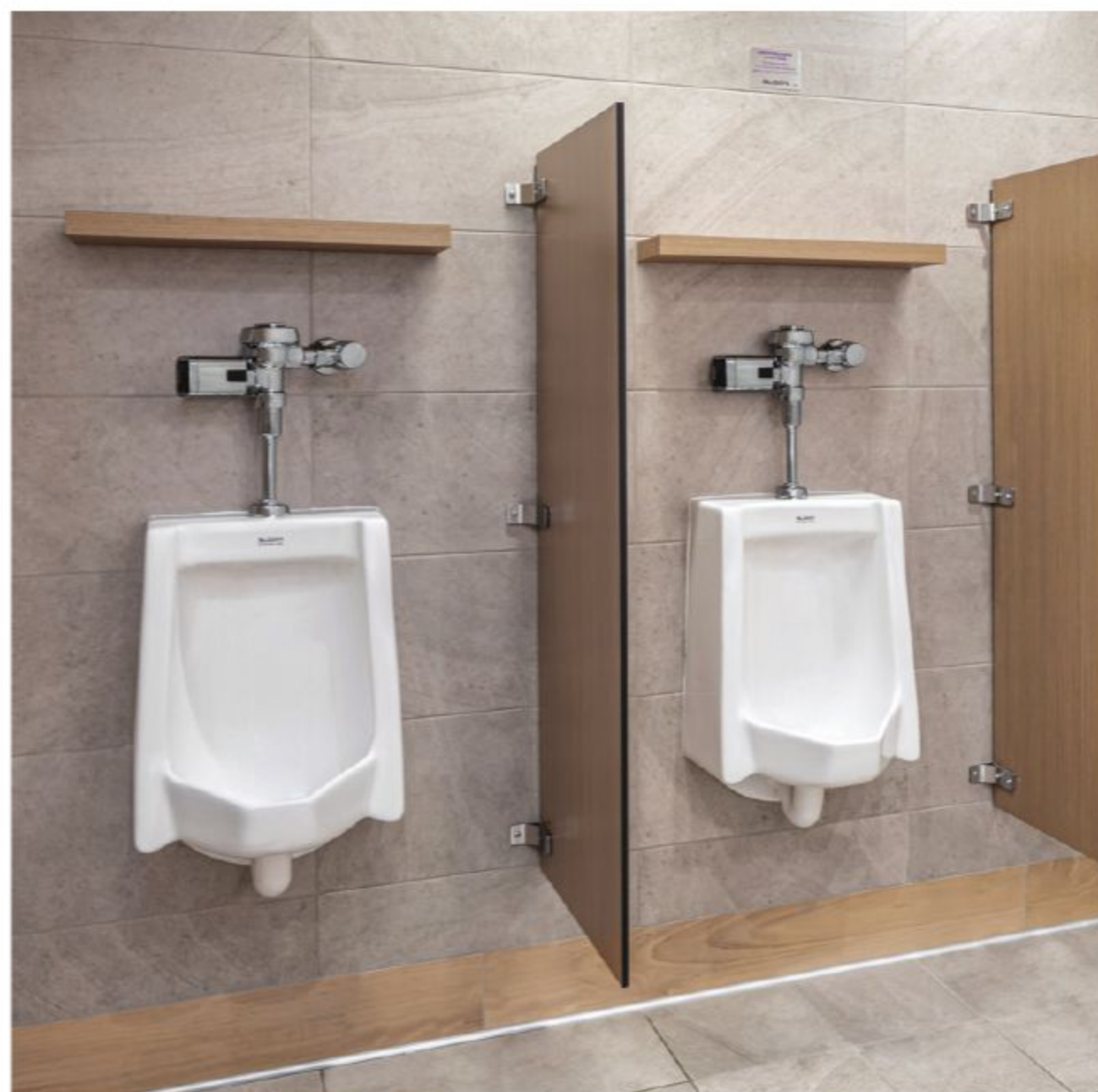
Sensor flushometers, equipped with reclaimed water features, are designed to withstand the harsh conditions presented by reclaimed water while conserving water at the same time.
